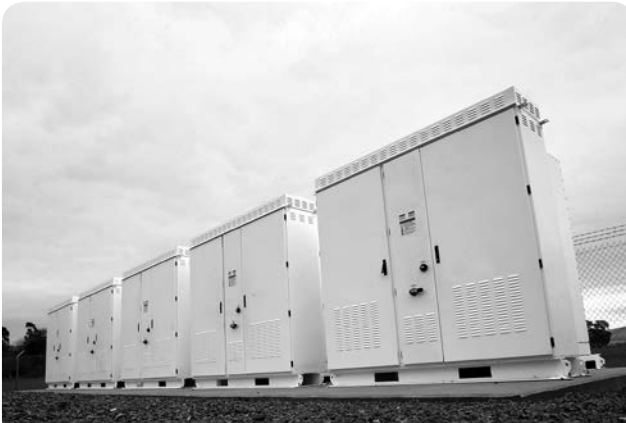
Tesla's battery storage facility can store a megawatt of alternative energy, allowing the district to use more 'green' power during peak times of the day.
