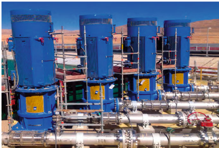
Fig. 3 Vertical turbine pumps made from reused parts in Chile. Source: Neptuno Pumps (2018)
