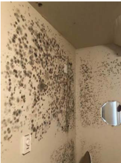
Figure 3.16 Large area of fungal growth on walls. Wet building materials provide excellent growth media for mold. Source: Reproduced with kind permission of Martin Rose.
