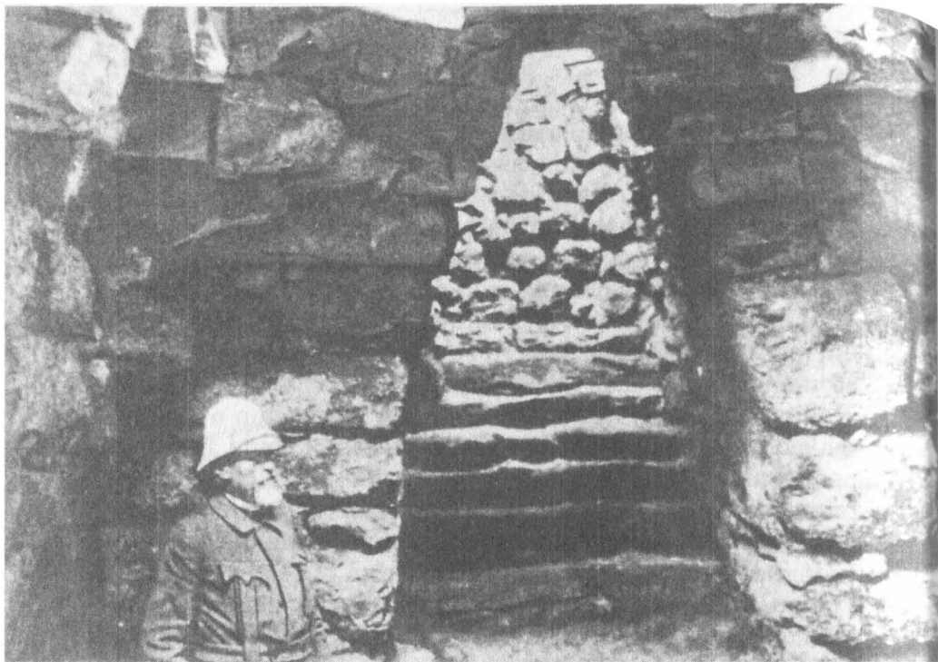
7.25 A built tomb at Megiddo, roofed in the corbeling technique. This large tomb, found close to the Canaanite palace, may have been a royal burial place. Schumacher, the excavator of Megiddo between 1903 and 1905, is seen in this old picture.
